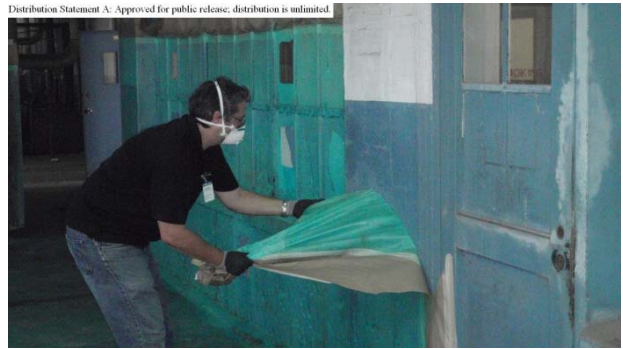
Figure 13. Dried DG can be easily peeled off from a variety of surfaces including bare concrete, three dimensional control panels and equipment, windows and walls.
