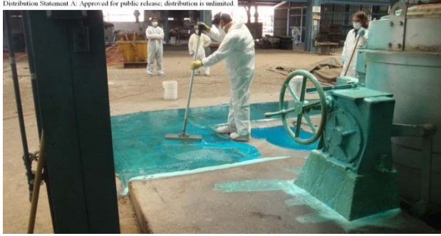
Figure 11. Application of DG (1101) by trowel (left photo) and brush (right photo).
