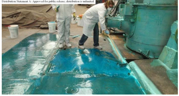
Figure 11. Application of DG (1101) by trowel (left photo) and brush (right photo).
