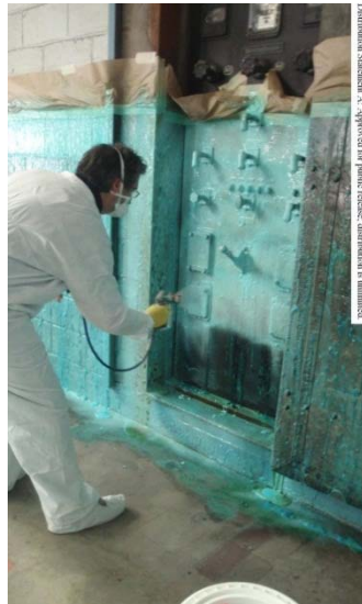
Figure 10. Sampling before decontamination and application of DG (1121) by spraying on vertical and three-dimensional surfaces.
