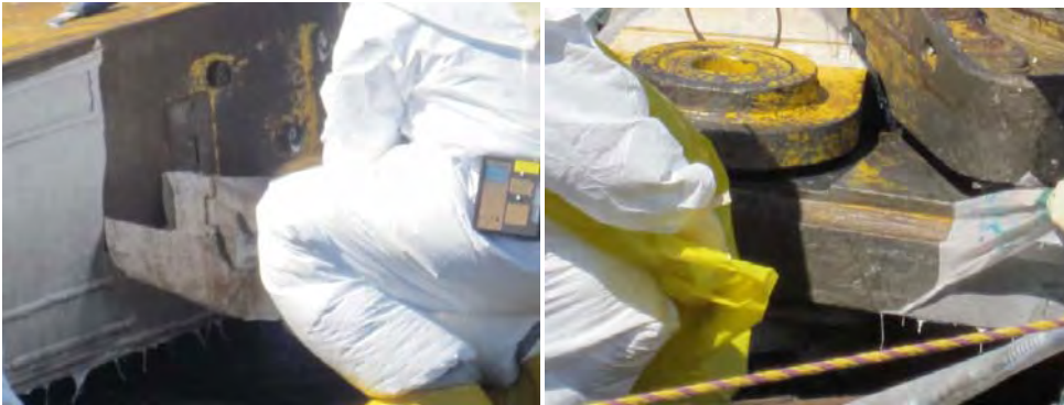
Figure 5 – Application of DeconGel 1101 & 1121 on contaminated excavator sheers.
