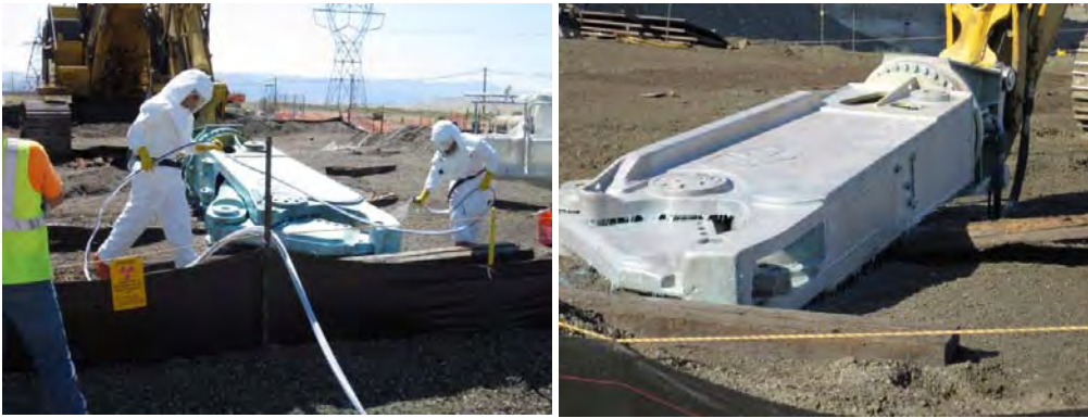
Figure 5 – Application of DeconGel 1101 & 1121 on contaminated excavator sheers.
