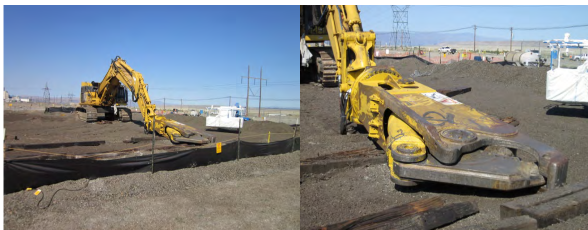
Figure 4 – Kamatsu 800 Excavator Shears used in demolition of 100KE Basin.
