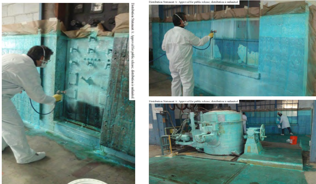
Figure 10 – Application of DeconGel 1121 by spraying vertical and three-dimensional surfaces.
