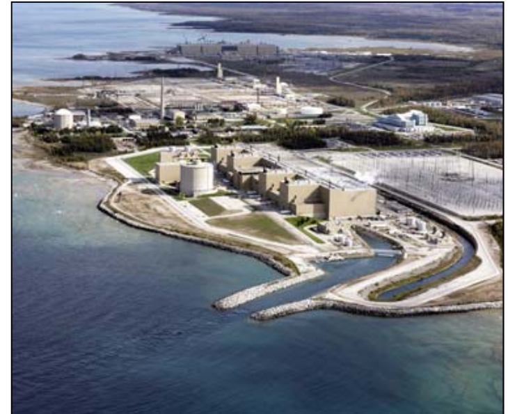
Bruce Nuclear Generating Station Ontario, CA
